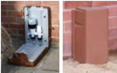
Wall mount box in situ and insuduct
